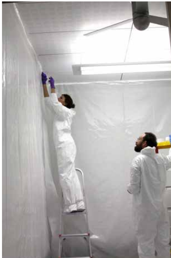
Microbiologists Jessica Green and James Meadow of the University of Oregon’s Biology and the Built Environment Center seal a room in preparation for an experiment measuring how human occupancy alters the microbial profile of inhabited spaces. (PHOTO: ANGIE PONSO)
